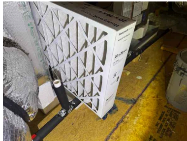
Filter Location: Air Handler Equipment, Fresh Air Filter
