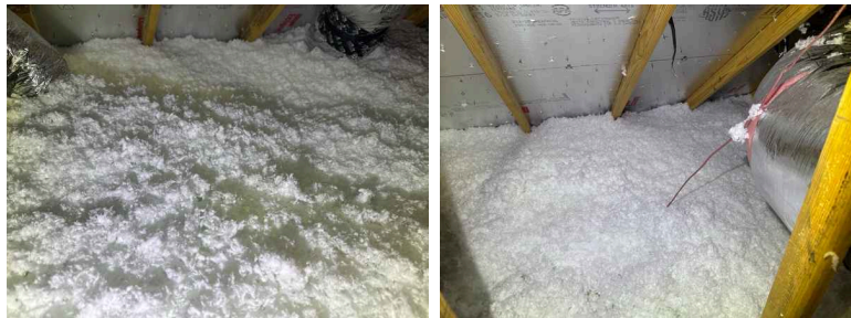
Type of Roof Decking: Radiant Barrier, OSB
