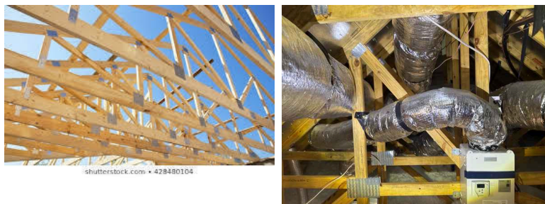
Type of Roof Structure: Engineered Trusses
