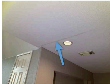
2nd Floor hallway
