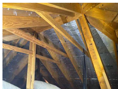
Type of Roof Structure: Conventional Stick Framing
