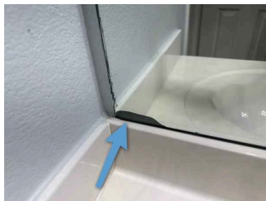
2nd Floor Bathroom
