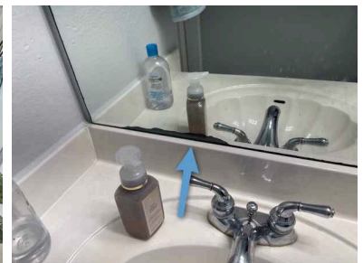
2nd Floor Bathroom
