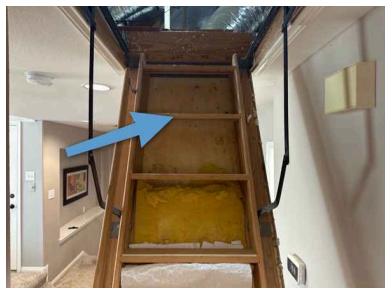
2nd Floor Attic
