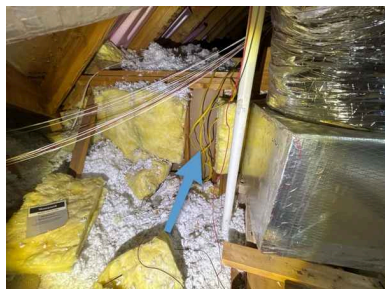
2nd Floor Attic
