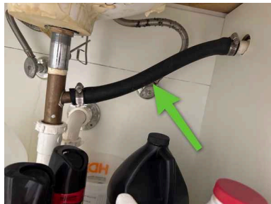
2nd Floor Bathroom
