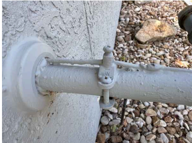
Type of Gas Distribution Piping Material: CSST, Black Metal Pipe Comments:
